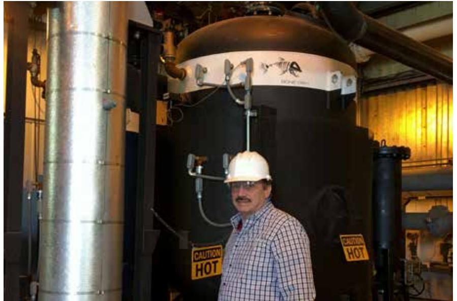
Norm Fischer chief engineer of The Fischer Group. Norm designed a new high-tech way to remove humidity and contaminants from the air, a necessity for industrial manufacturing.
