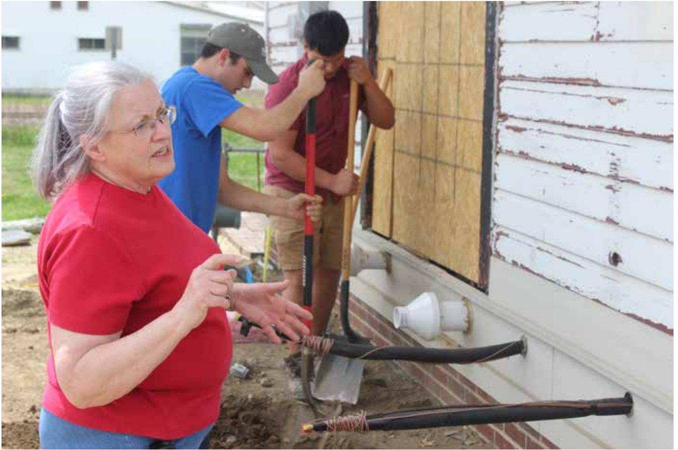
Former construction field project manager, Barbara Biernat, left her career to lead the building trades program at the Porter County Career and Technical Center. She and her students are renovating a 1912 train depot at the school's campus. Once completed, it will be used as a new school of cosmetology for the career center.
