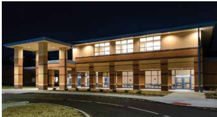
Photo provided by Larson-Danielson Construction
